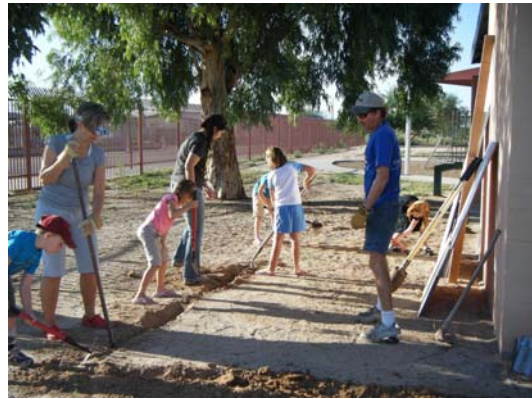
Building the chicken coop.
